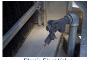
Plastic Float Valve Replaced with Marley Brass Valve
