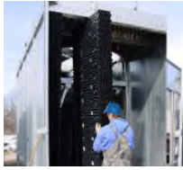
Fill Replacement Hanging fill & Bottom Supported
