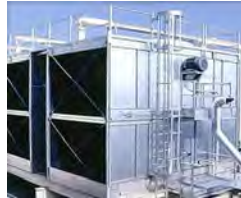
Tower Access – Safety Equipment
